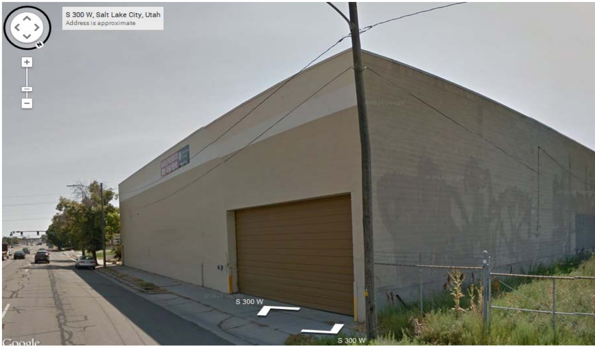
The east portion of the existing building that fronts on 300 West
